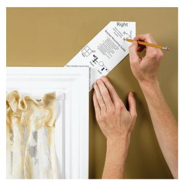
Step One: Using the Bracket Mounting Template shown above, mark the location on the wall for the mounting screws.
