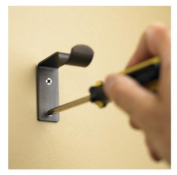
Step Two: Drill two pilot holes per side for each bracket (3/16" drill bit) insert wall anchors and attach to wall with screws provided.
